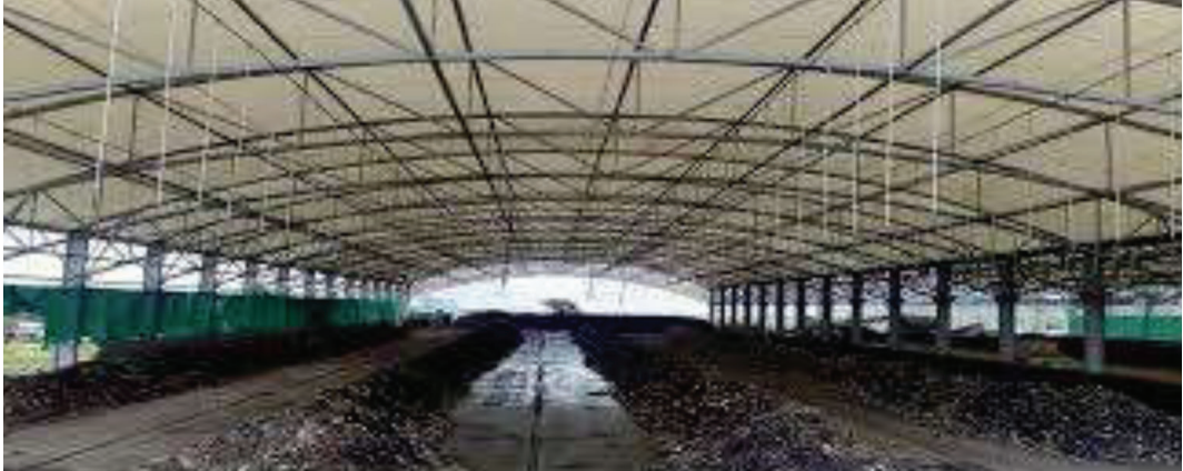
VINDROW COMPOST PLANT
