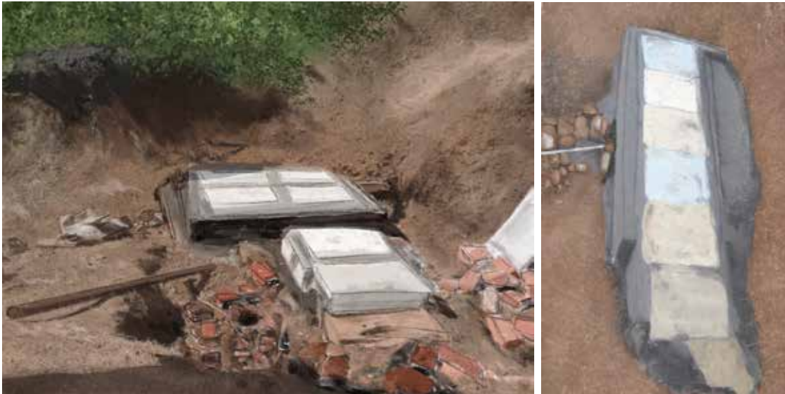
Figure 8.16: (a) Spring Box with open bottom (b) Spring Box with open side
