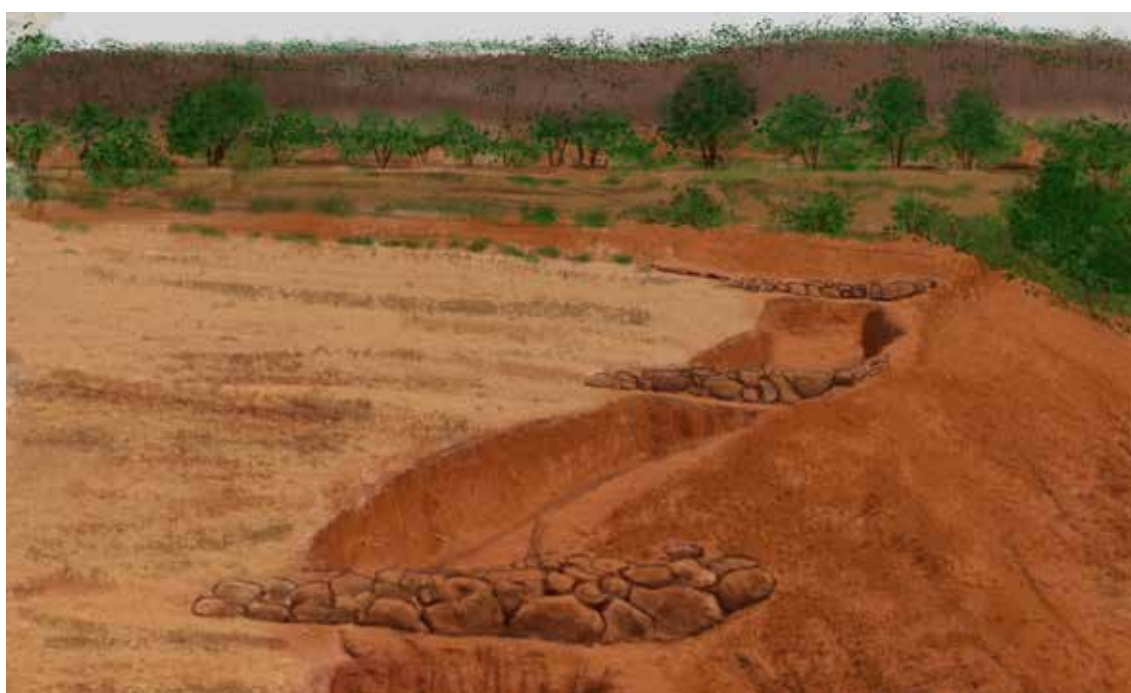
Figure 8.7: An earthen contour bund on slope that is > 10%
