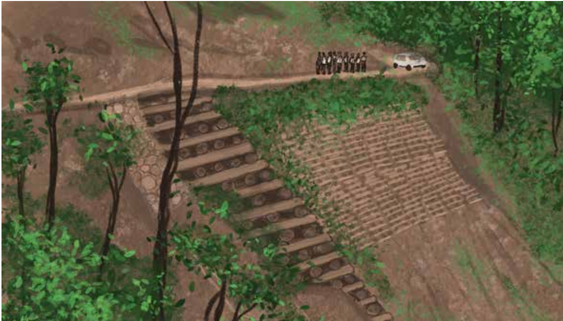
Figure 5.10: Timber crib wall with quick-set live cuttings
