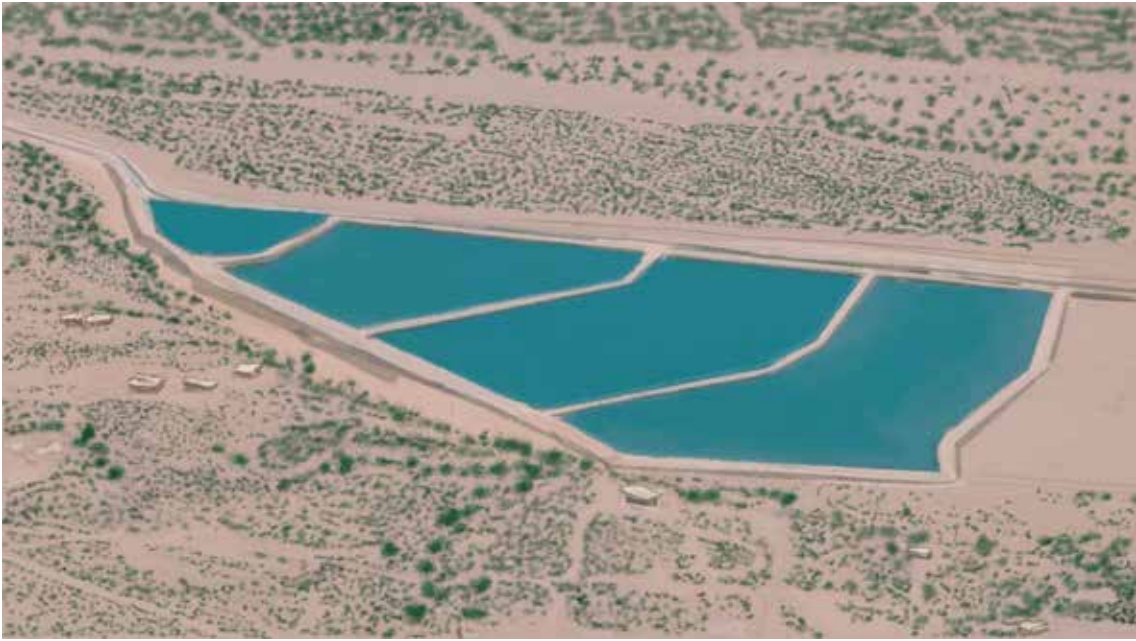
Figure 8.24: Flood water spreading system on a cascading water basin for MAR
