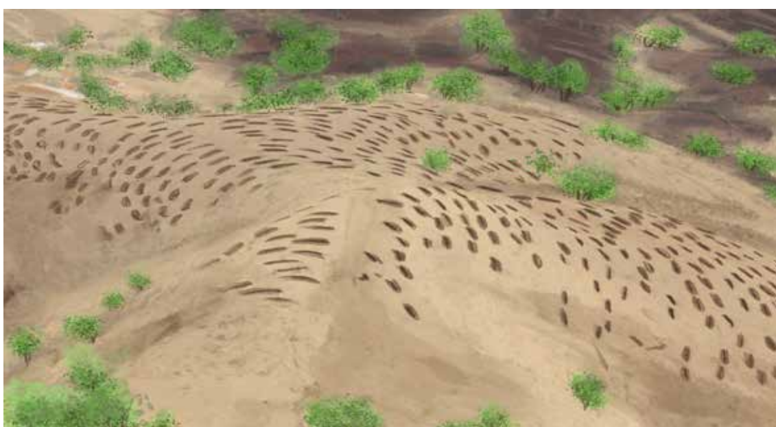
Figure 8.3: Staggered contour trenches along the lopt to check the velocity of surface runoff & soil erosion
