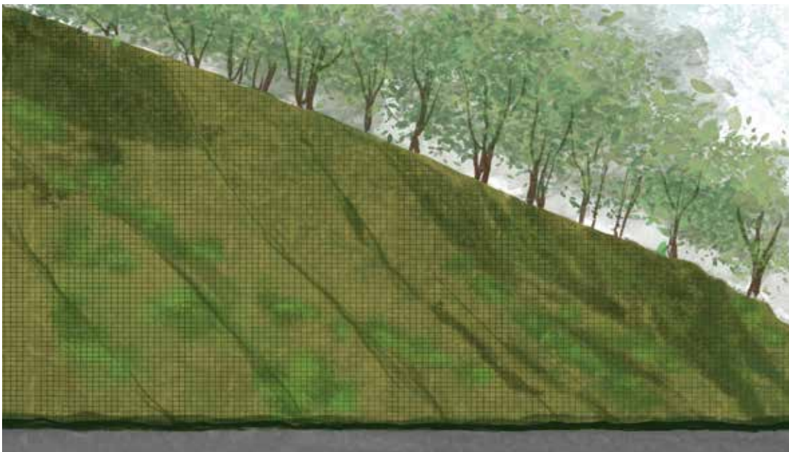
Figure 5.7: Slopes stabilized with biodegradable geotextiles in Hong Kong
