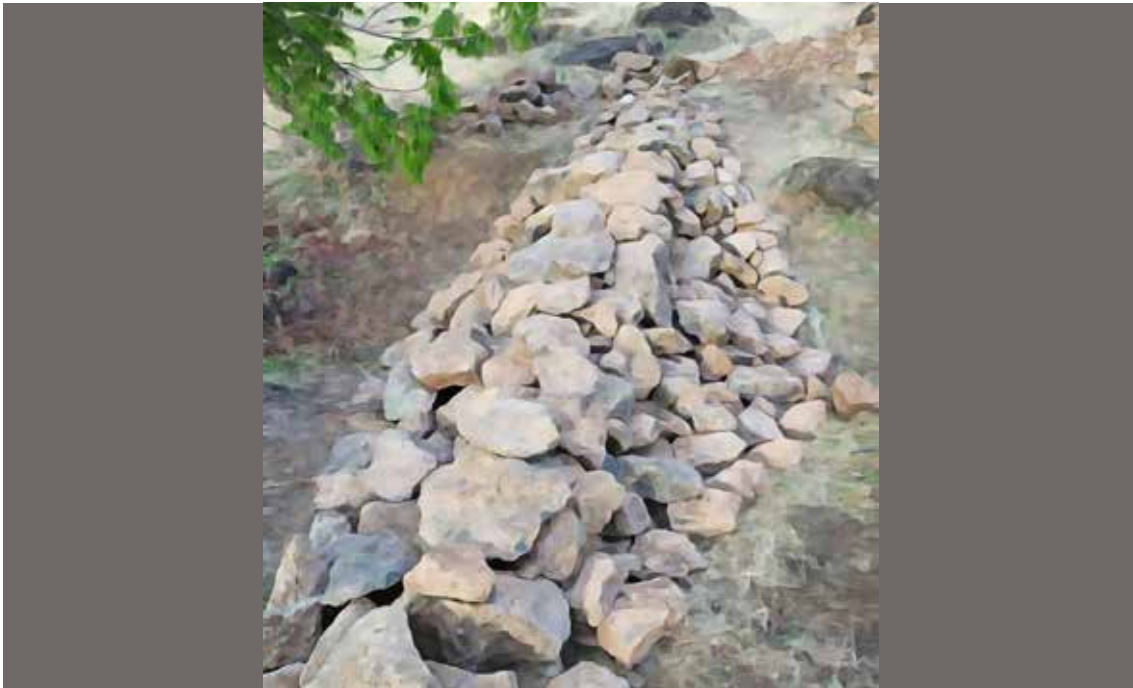
Figure 8.11: A LBS constructed along an ephemeral first order stream
